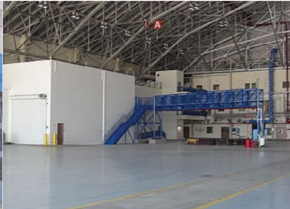
The skywalk will afford access to the plane's port side; next to it (and also new) are two high-bay rooms for mirror stripping and mirror coating. Yellow lines in foreground mark the center taxi line for the aircraft.
