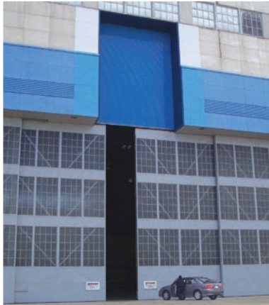
Tail cut out above the massive doors allows the 747SP's 65-foot high vertical stabilizer to enter the hangar. It is one of several major investments by NASA to tailor N211 for SOFIA .
